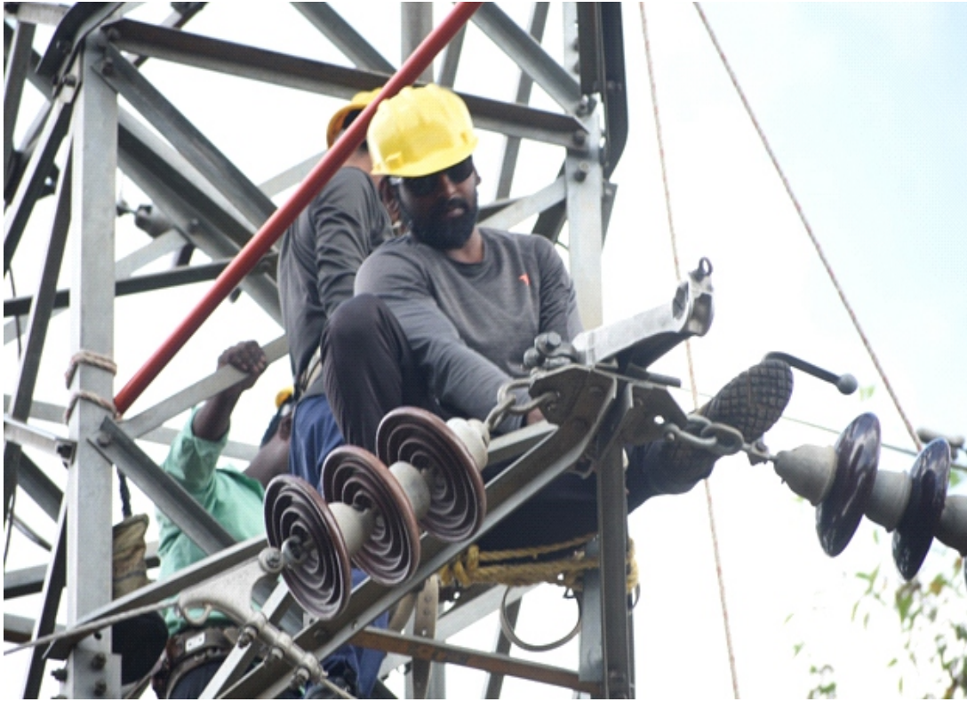
Back end yoke fitting work
