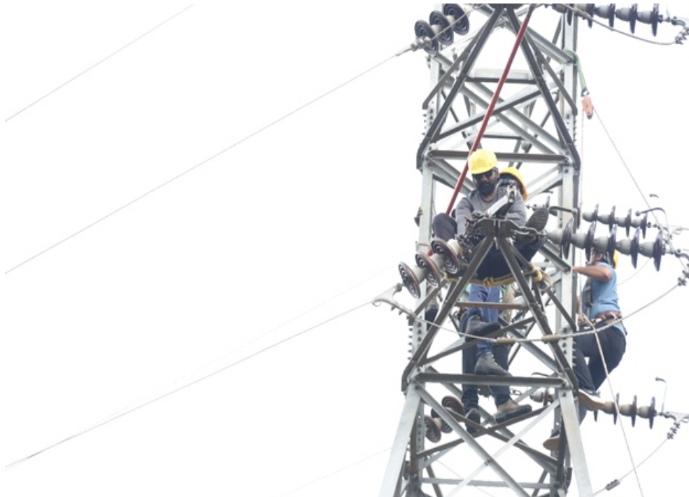
66kv tension insulator replacement work
